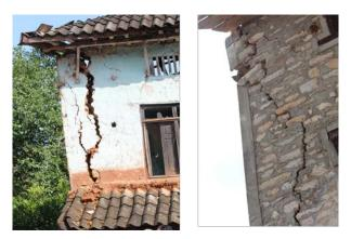
Figure 4. Separation of walls in corners where horizontal bands were absent
