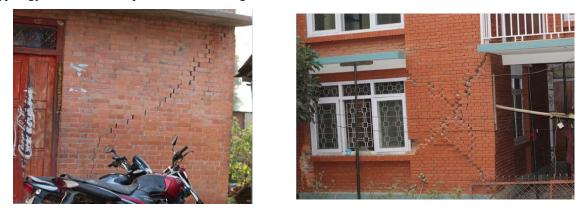
Figure 5. Diagonal in-plane shear cracks in brick masonry walls
