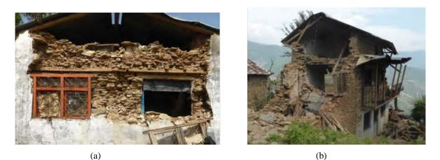
Figure 3. Out-of-plane failure of walls in stone masonry houses: (a) delamination, (b) complete failure of walls
